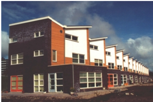
figure 1 – View on the rear side of the energyneutral homes Pieter Christiaanpark, Leeuwarden.
